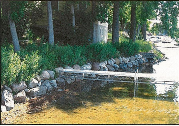
Shrubby vegetation planted above a rock toe prevents erosion better than grass or a lawn especially in circumstances of flooding and intense wave or ice action.
